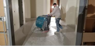
On Left: Terrazzo floor in the hallway between the Library and the Theater receiving its first grinding. Later it will be finely polished and sealed.
