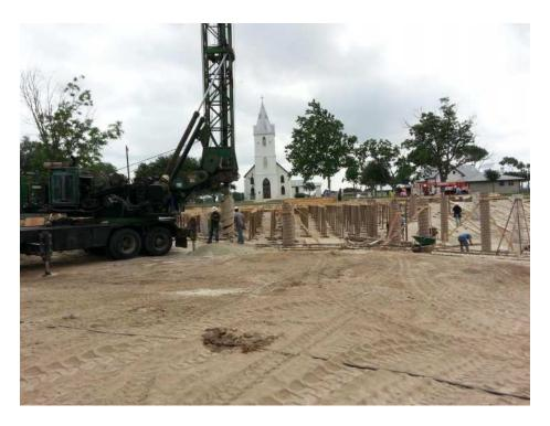
Continuation of drilling of the piers and the construction of the form for the foundation, Week 5
